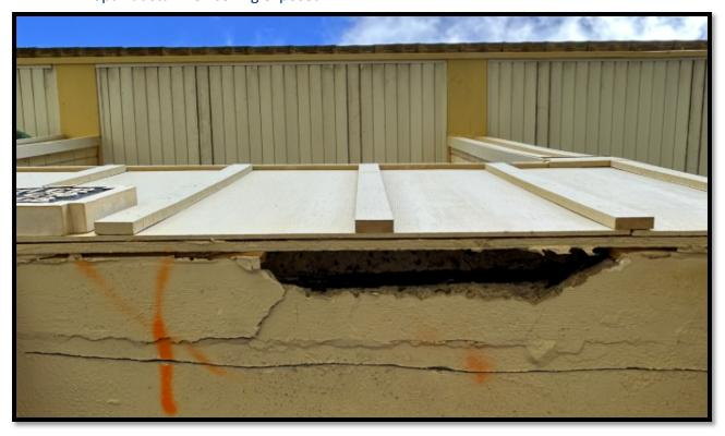
• Spall at stairwell end wall exposed
