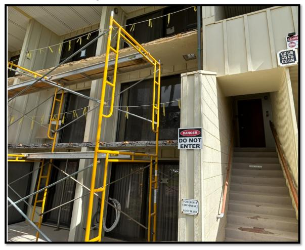
• Leading edge of 3<sup>rd</sup> floor lanai demolished
